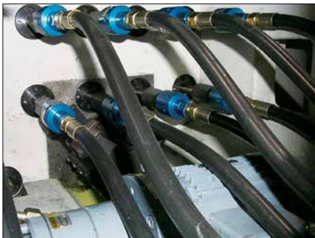
DEUBLIN 1116 Bearing-Supported Unions on Automotive Transfer Line
